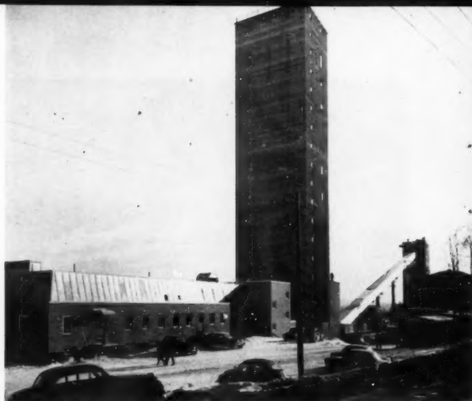
MINE AND MILL PLANT with change house, concrete headframe and secondary crushing, ore conveyor, and the concentrator building. Note clean functional lines of buildings.
